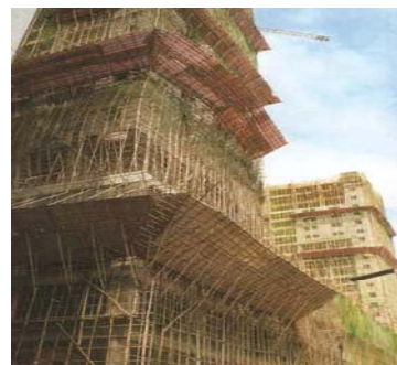
Fig. 6 Bamboo canes used for scaffoldings
