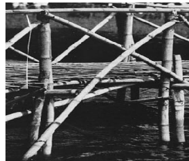
Fig. 11: Bamboo bridge with intermediate posts in the river bed
